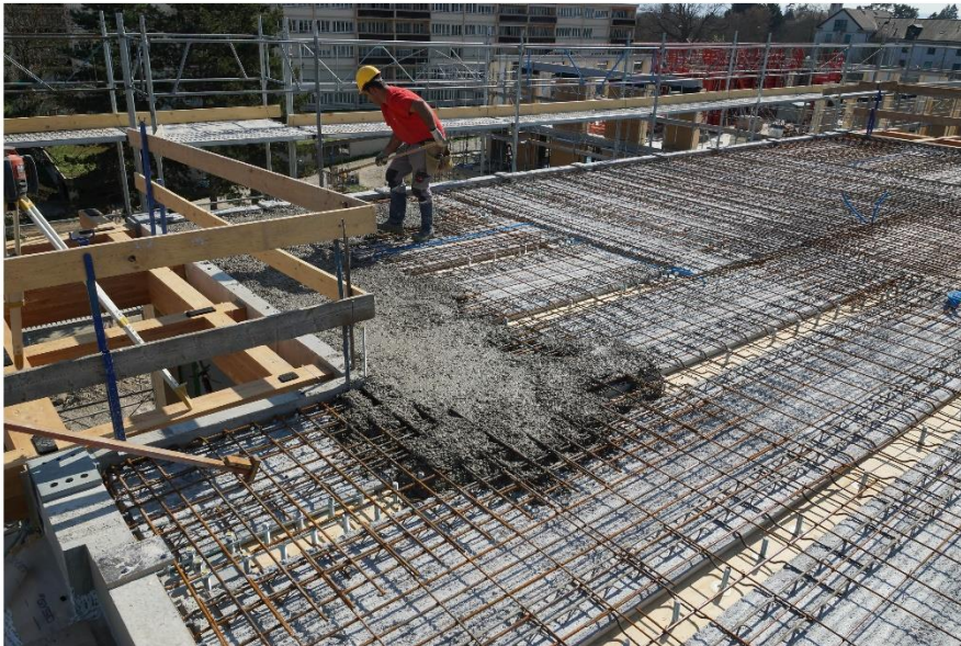
VIEW OF CONCRETE TOPPING
