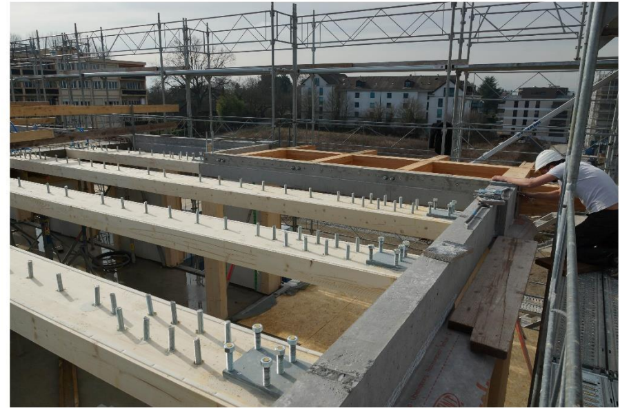
VIEW OF THE ASSEMBLY CONCRETE BEAM AND GLULAM BEAM
