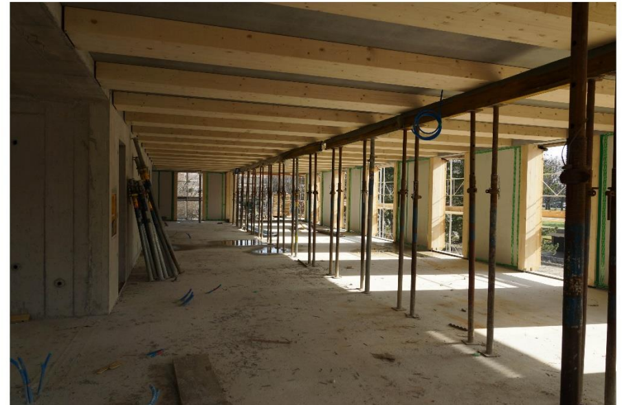
VIEW ② GLUED LAMINATED BEAM
